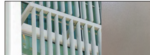
LV1: NICKEL PEARL POWDER COATED ALUMINIUM AEROFOIL LOUVRES LRV: 48%
